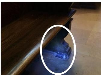
In the photo above, custom-made 1/8 inch brackets were designed to re-secure the pews to the travertine tile floor.
